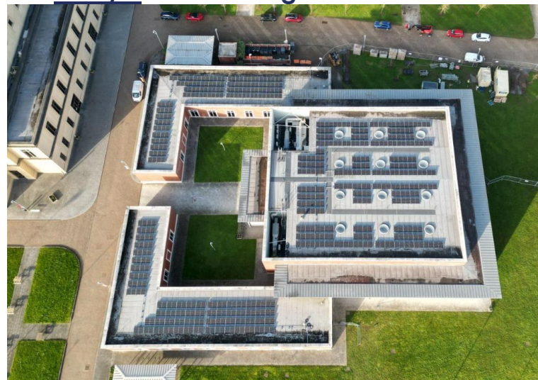
Bay Campus Library solar array
